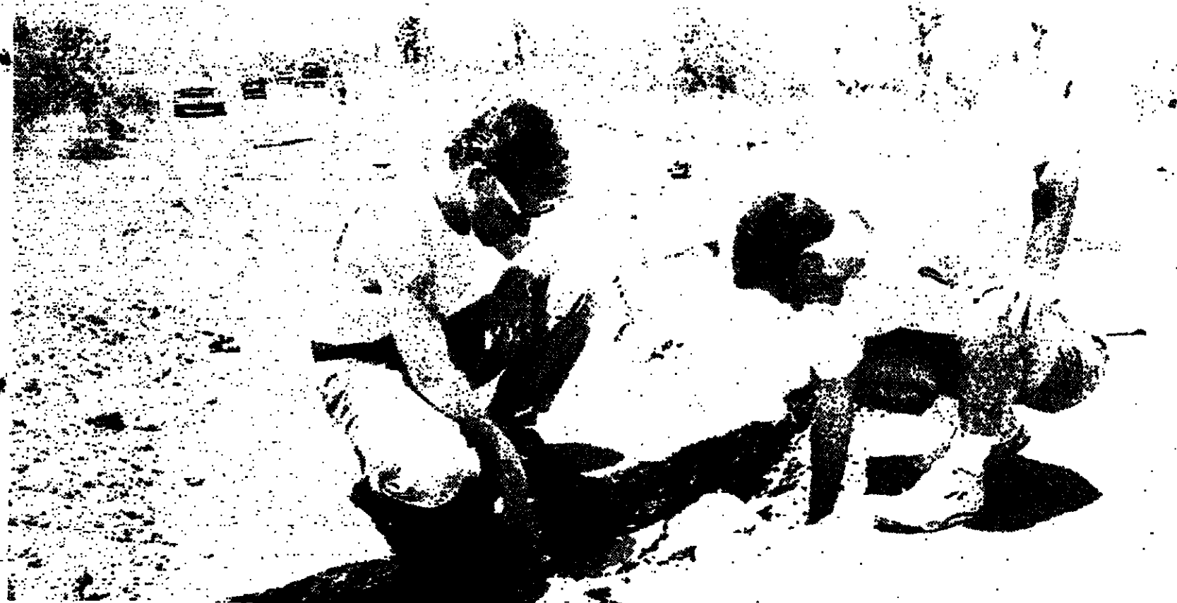
Two men taking a close look at a crack in a highway caused by one of the California earthquakes. Aftershocks hit California on Monday, causing skyscrapers to sway.
